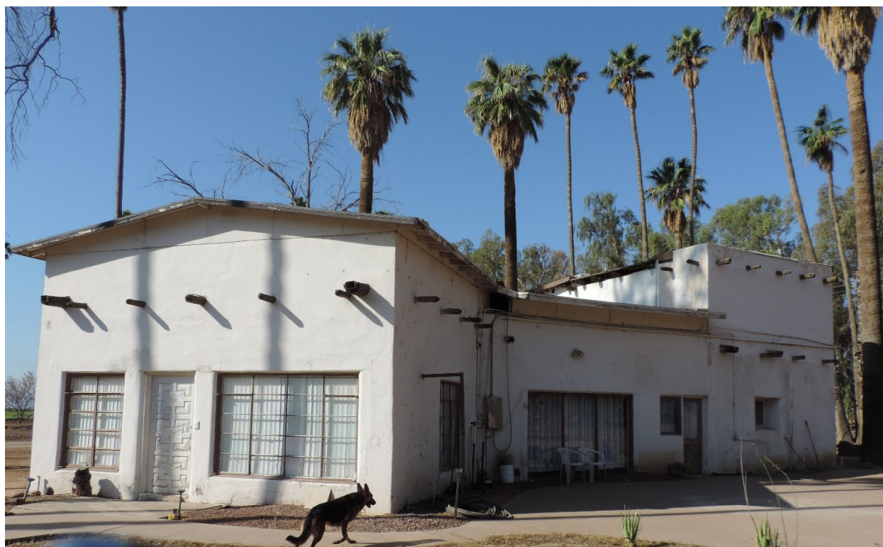
Photo 1. 1930 Adobe residence, view facing southwest. (Karen Krause photo, August 2023)
