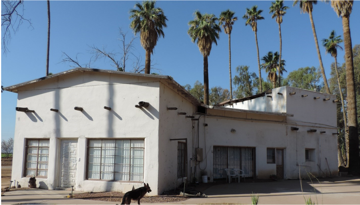
Photo 1. 1930 Adobe residence, view facing southwest. (Karen Krause photo, August 2023.)
