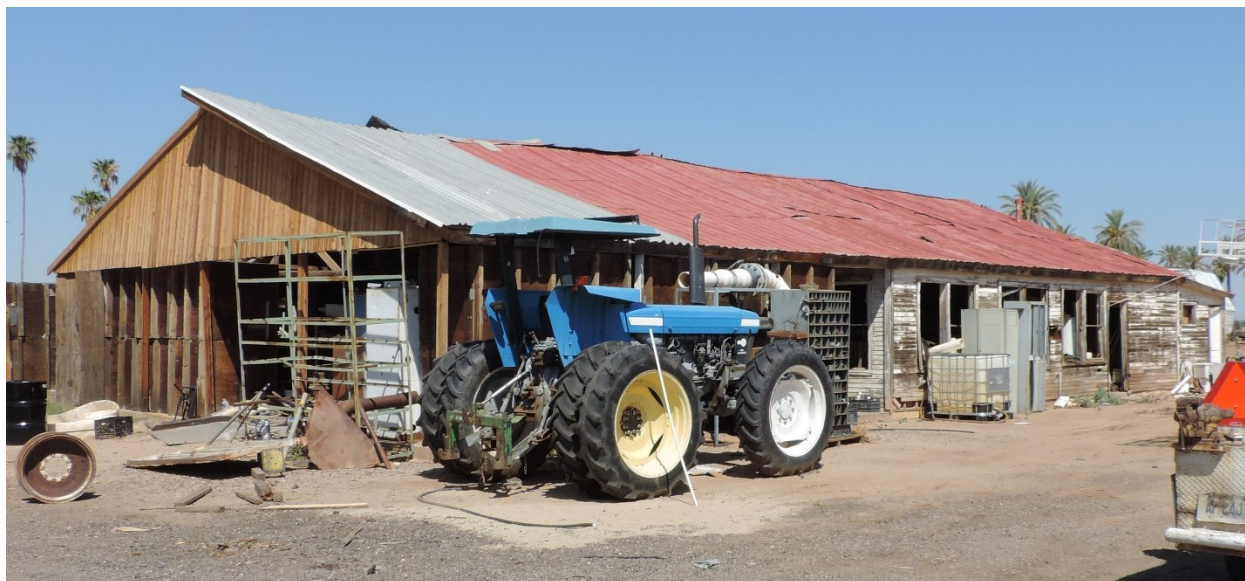
Photo 16. South and east elevations of the old packing building. View facing northwest. (Karen Krause photo, August 2023)
