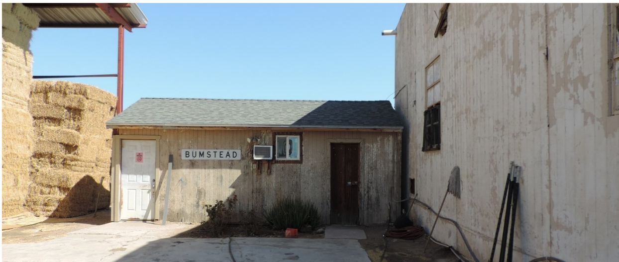
Photo 9. South elevation of the Shower and Toilet building to the west of the packing building. View facing north. (Karen Krause photo, August 2023)
