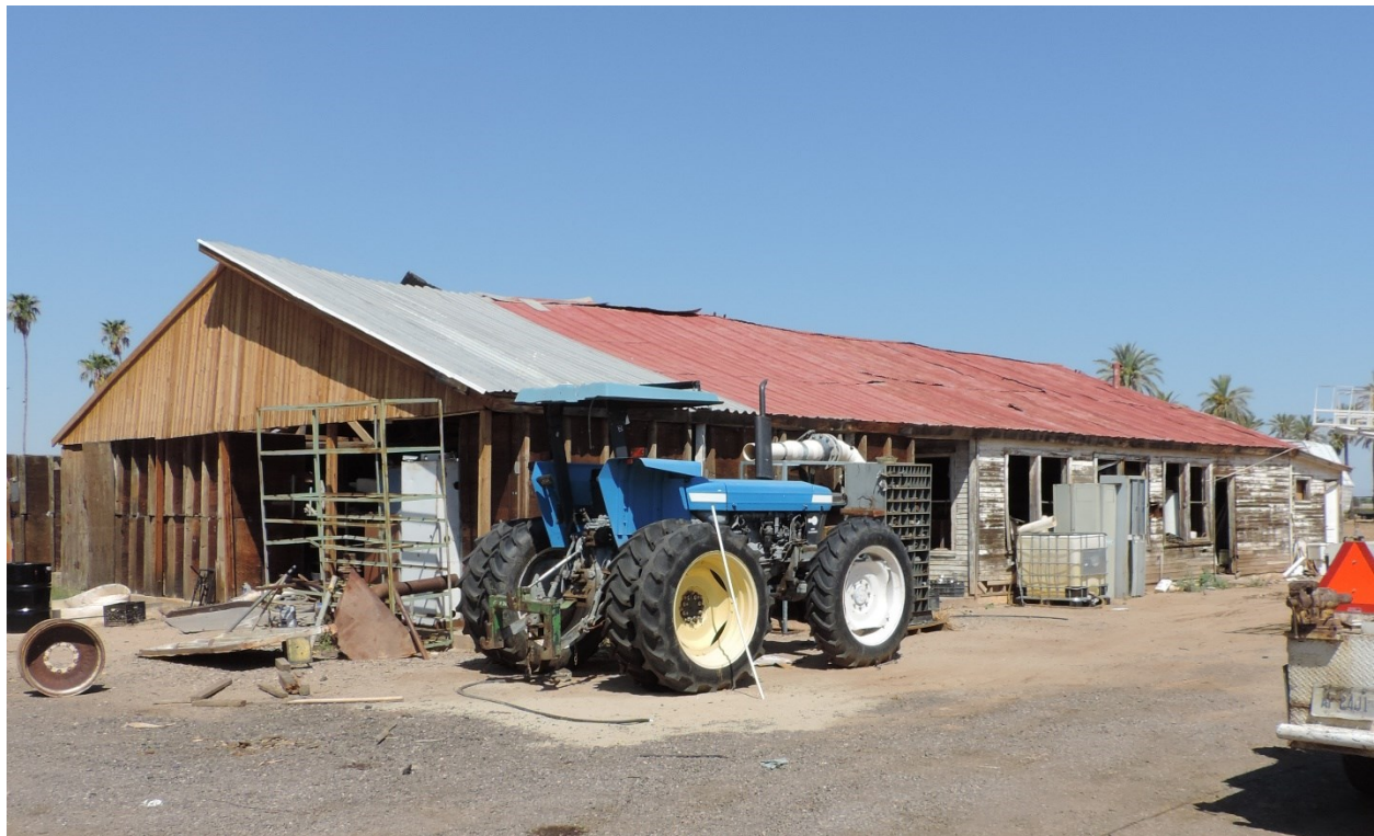
Photo 16. South and east elevations of the old packing building. View facing northwest. (Karen Krause photo, August 2023)
