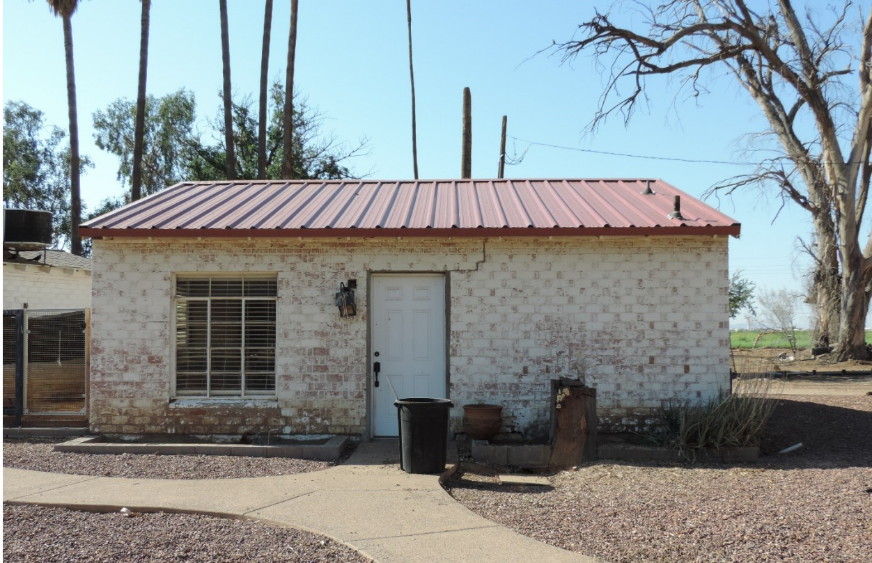
Photo 5. The north elevation of the housekeeper's house, built in 1946. View facing south. (Karen Krause photo, August 2023)
