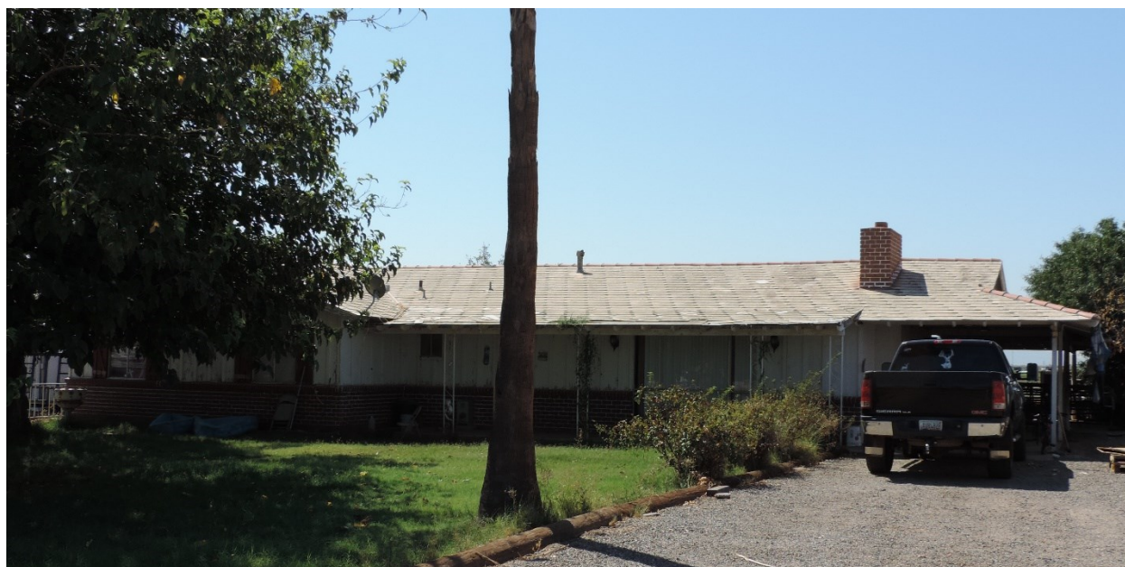
Photo 17. North elevation of the superintendent's house, view facing south. (Karen Krause photo, August 2023)
