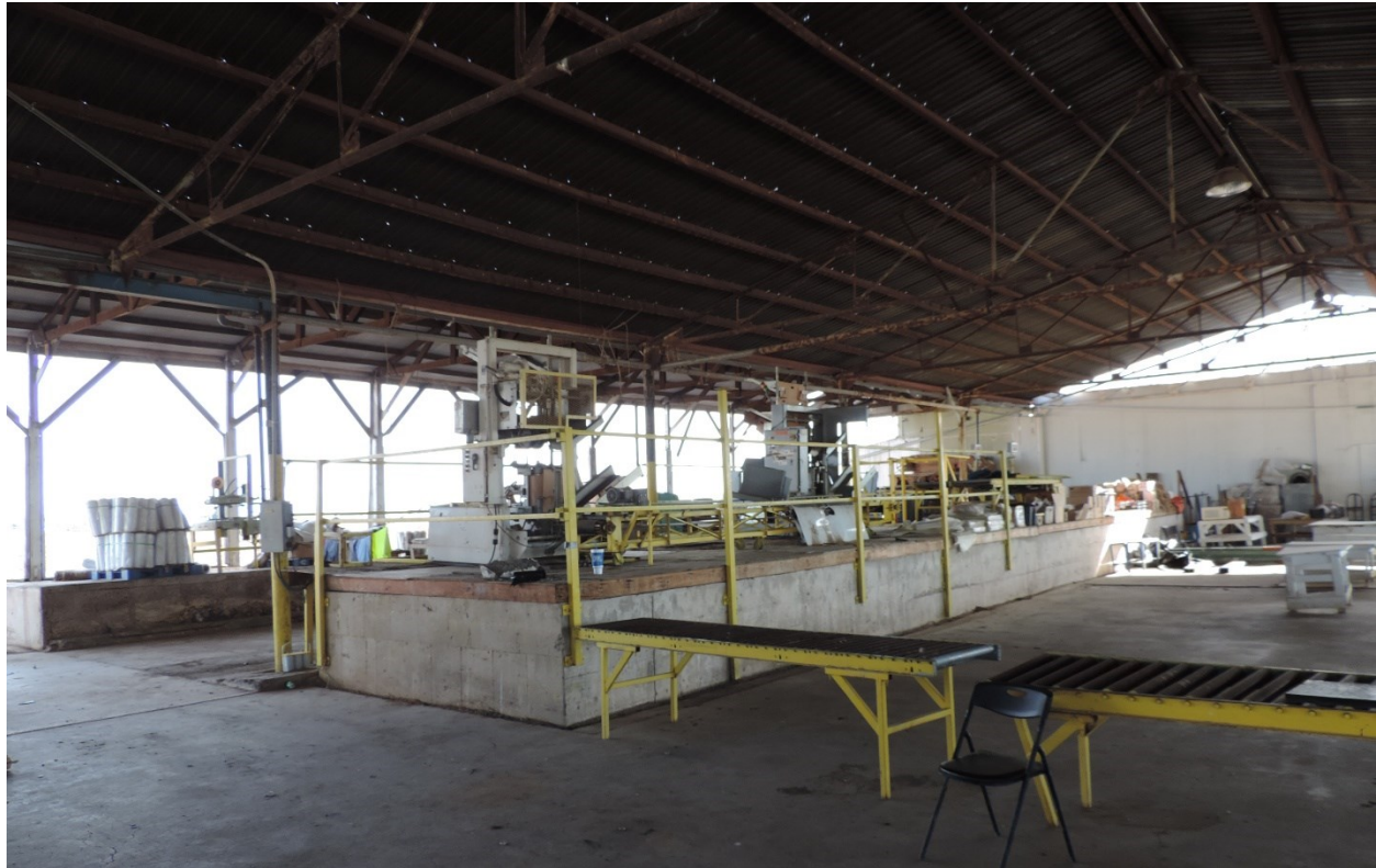
Photo 10. View of the loading dock and precooling tunnel and covered ice pit. View facing northeast. (Karen Krause photo, August 2023).
