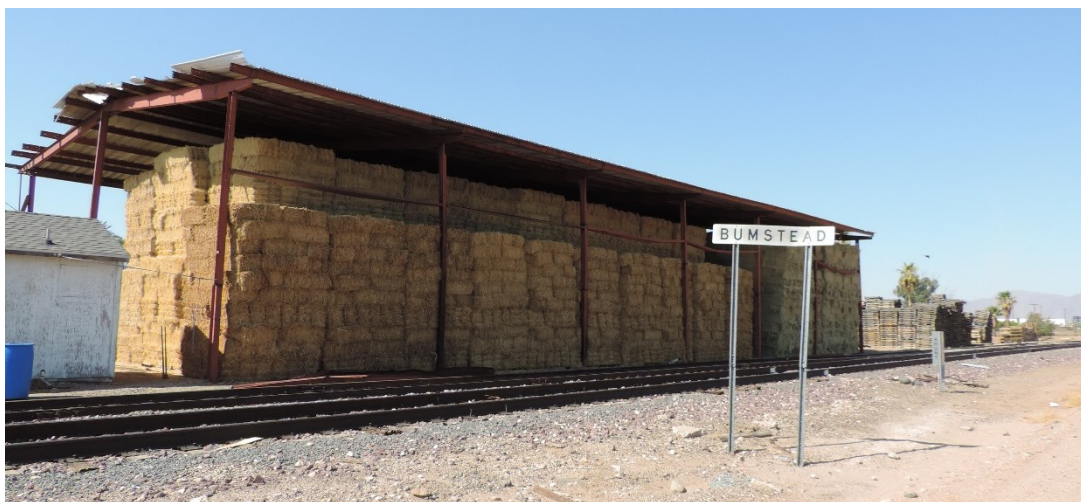
Photo 12. North and east elevations of the hay cover structure, the railroad, and the Bumstead siding. View facing southwest. (Karen Krause photo, August 2023)
