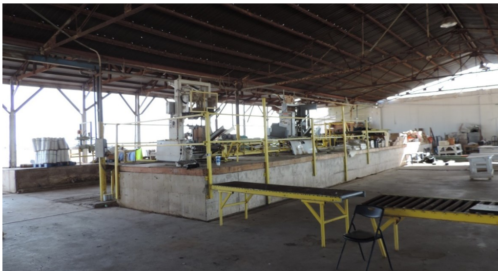
Photo 10. View of the loading dock and precooling tunnel and covered ice pit. View facing northeast. (Karen Krause photo, August 2023).
