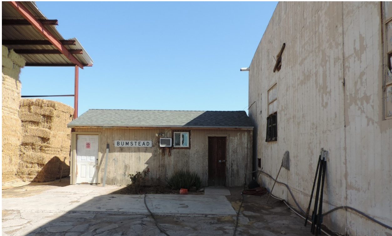
Photo 9. South elevation of the shower and toilet building to the west of the packing building. View facing north. (Karen Krause photo, August 2023)
