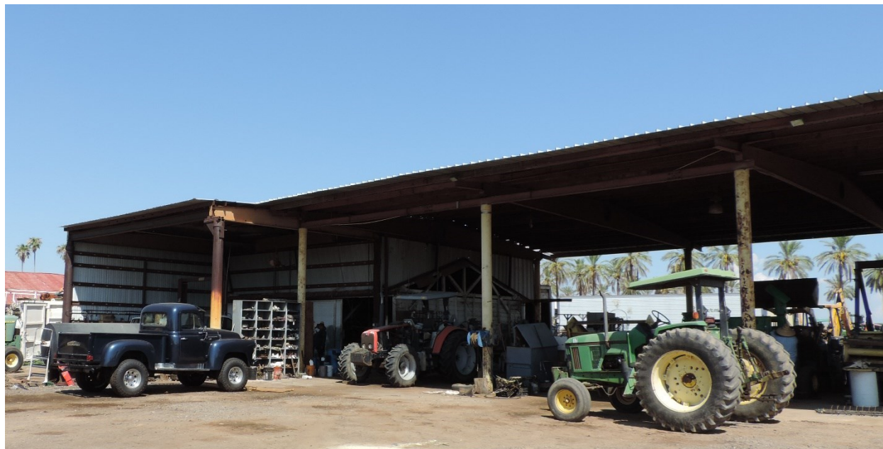
Photo 15. South elevation of the equipment shed as viewed facing northwest. (Karen Krause photo, August 2023)
