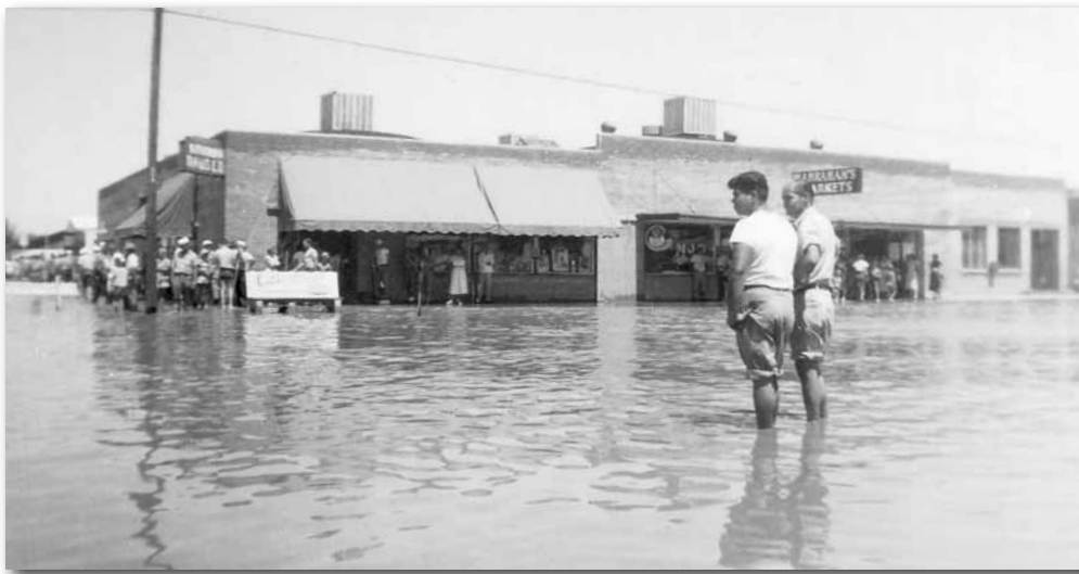
1951 flood. Businesses at Litchfield Road and Western Ave.
