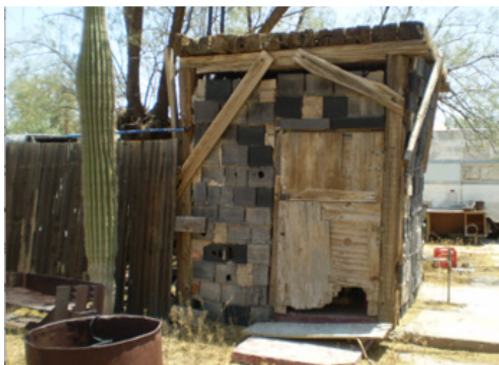
An outhouse made from old car batteries
